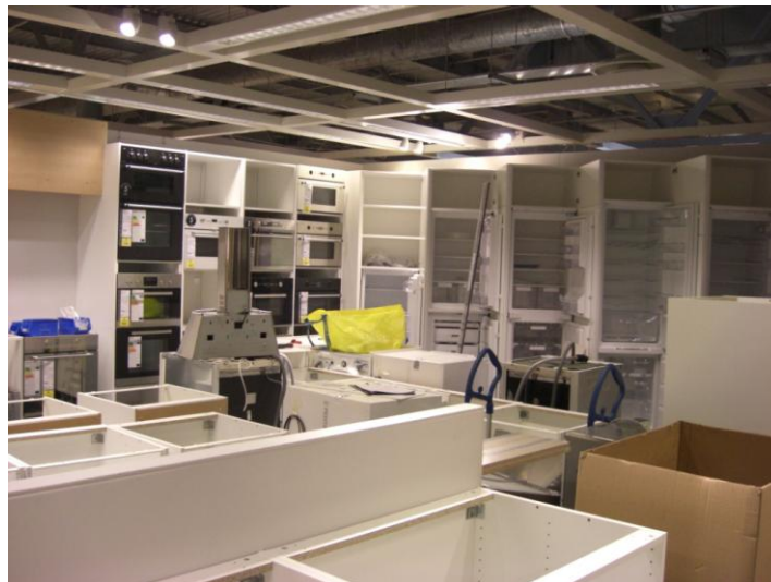
Figure. b1: Premise in the process of a refit.
